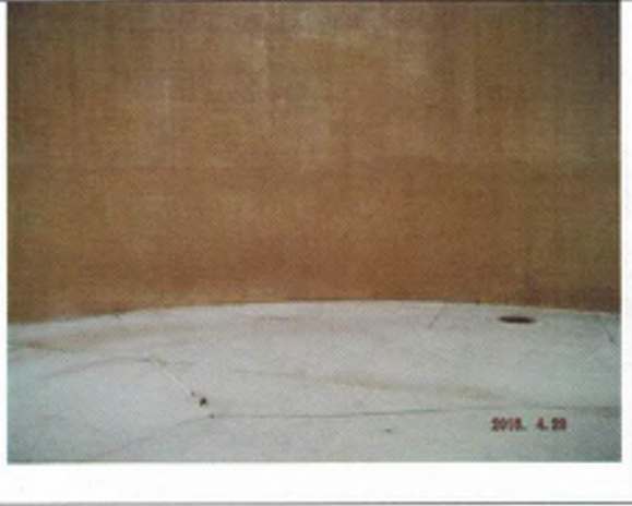
Interior sidewall and floor
