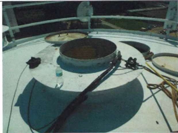
Access tube at exterior roof
