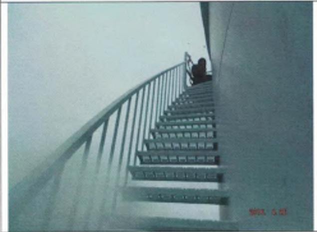
Upper sidewall staircase
