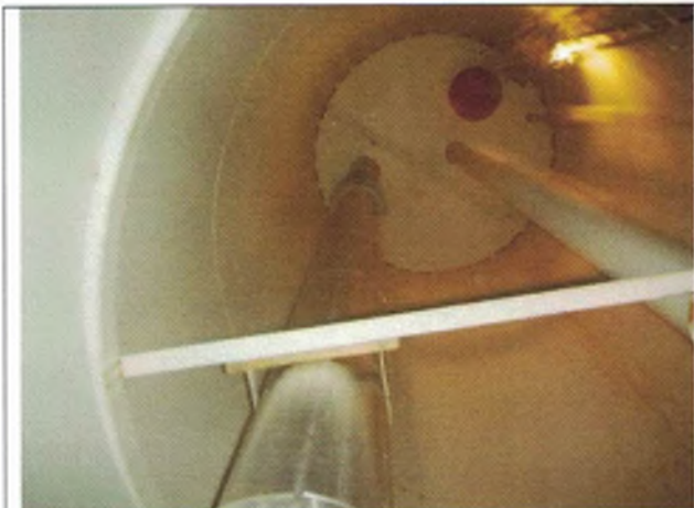
Looking up the interior pedestal
