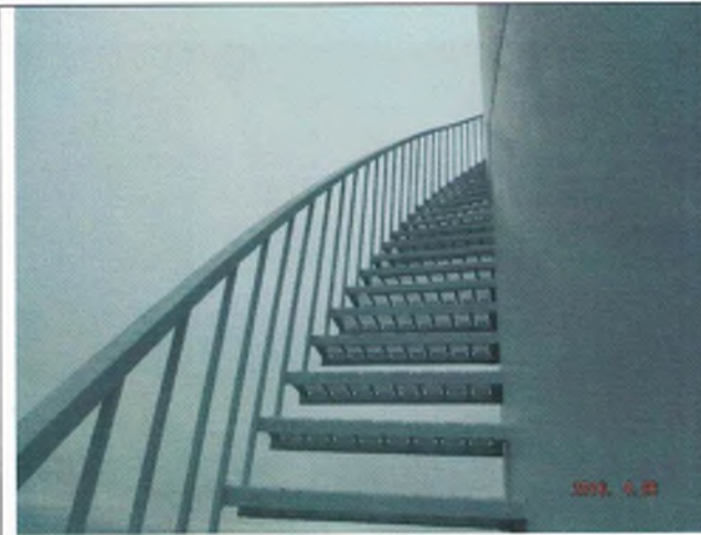
Mid sidewall staircase
