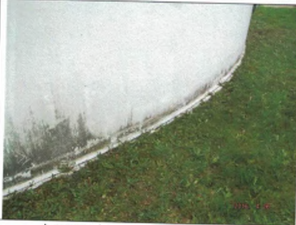
Lower sidewall and foundation
