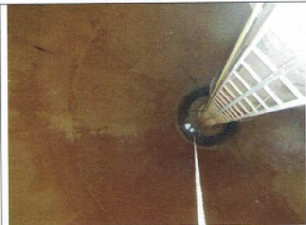
Looking down to bowl from roof
