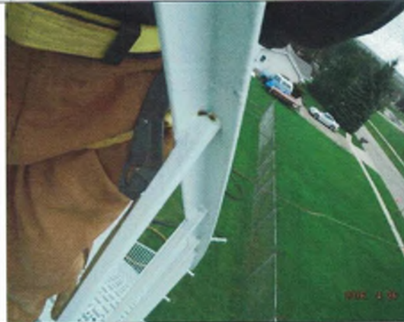
Typical view of bottom side of staircase handrail
