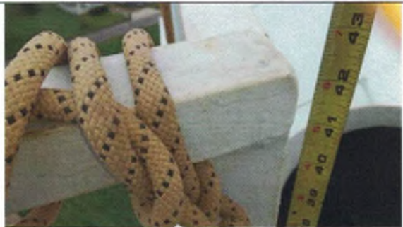
Roof handrail is 42" in height
