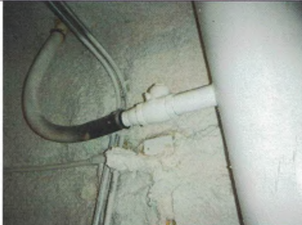
Condensate into the overflow
