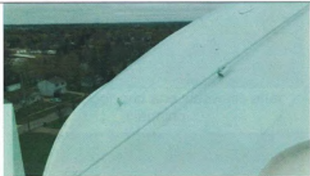
Exterior roof and obsolete conduit
