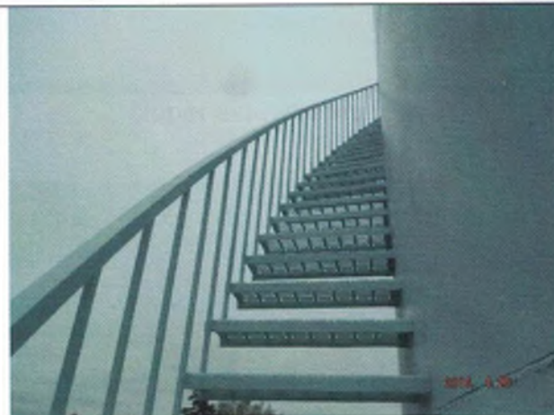
Lower sidewall staircase
