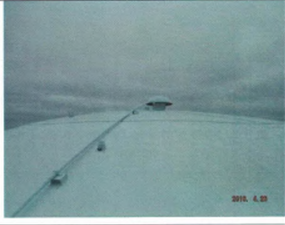
Exterior roof and roof vent
