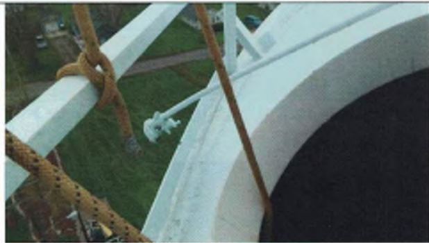
Cut off obsolete conduit on exterior roof
