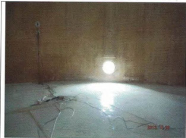
West hatch and floor
