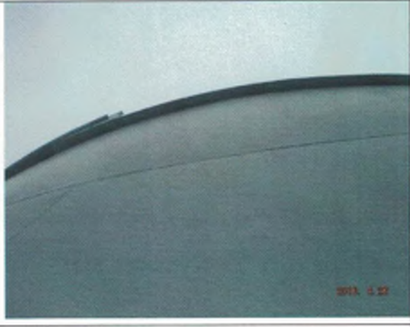
Upper exterior sidewall
