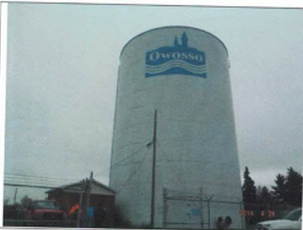
1,250,000 gallon standpipe, Owosso, MI
