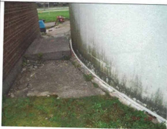
Lower sidewall and foundation
