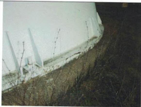
Baseplates and anchor bolts at foundation
