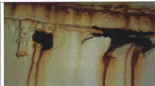
Close up of outer roof sidewall seam
