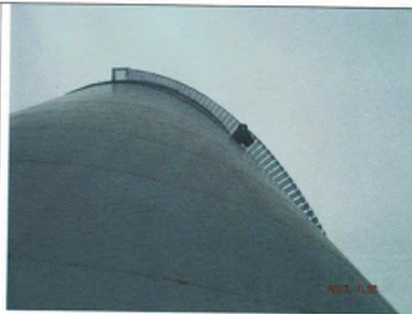
Exterior sidewall and staircase
