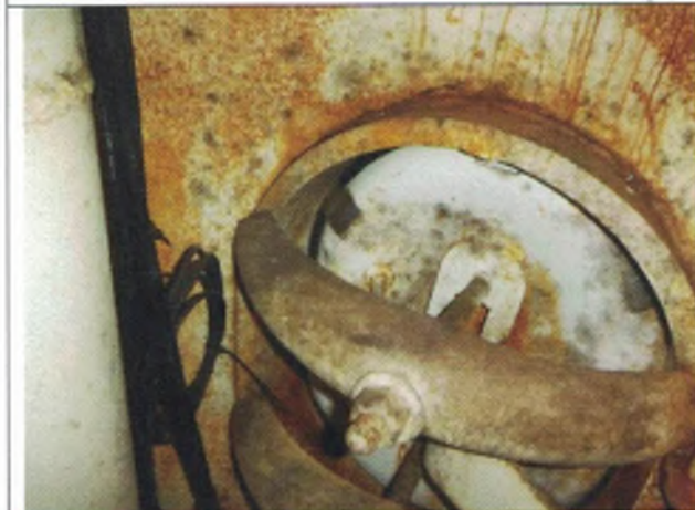
Dry interior access tube manway hatch
