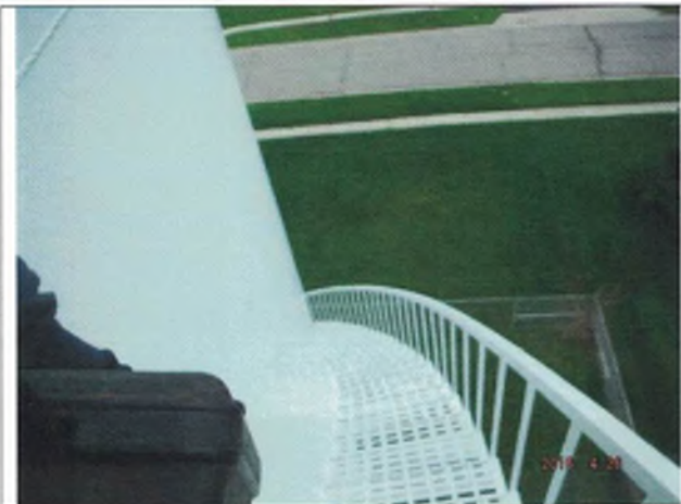
View of staircase from roof
