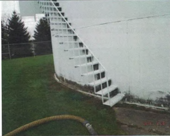
Lower exterior staircase
